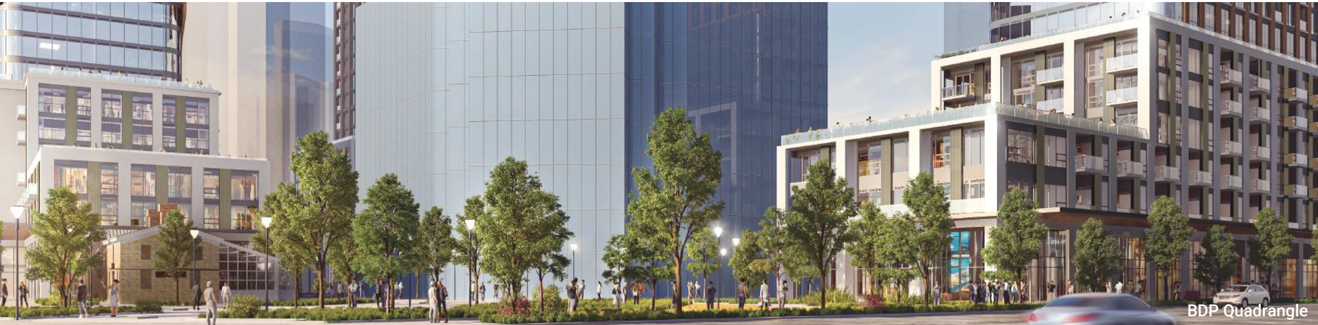
View of the POPS at the corner of Hurontario Street and Eglinton Avenue West
